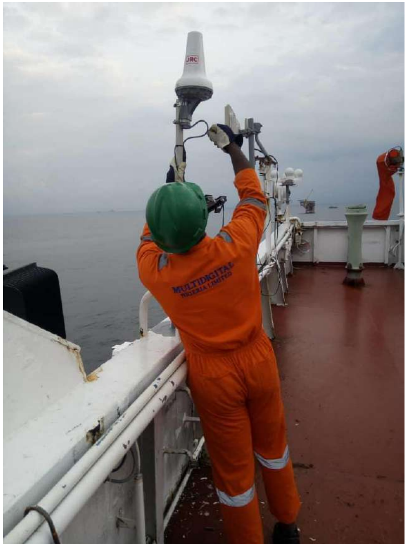
A Multidigital engineer repairs a JRC radar on a vessel
